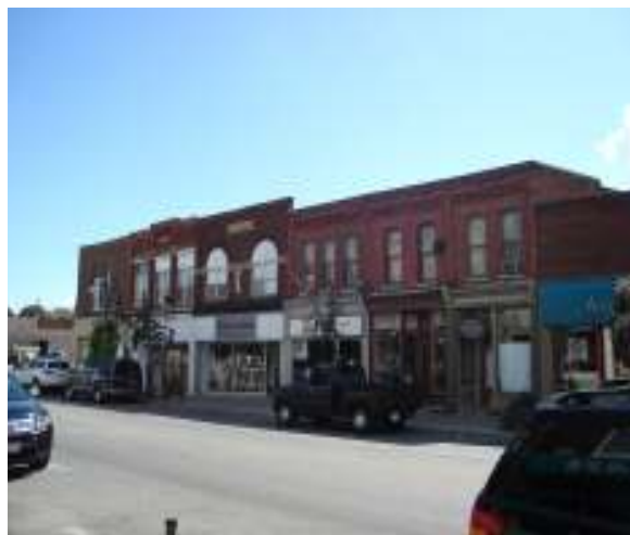
Talbot St East South side 2009
